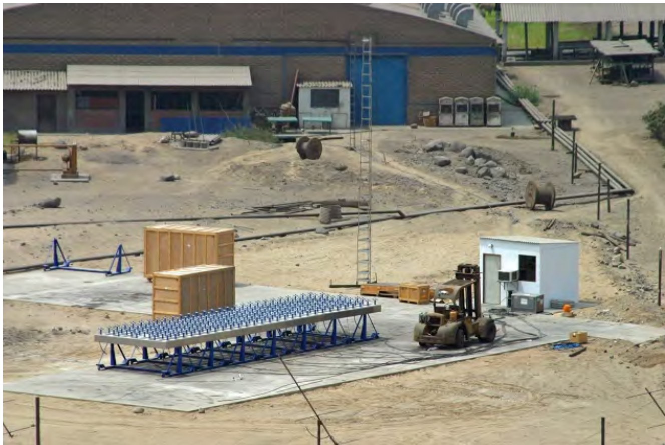
Seven AMISR panels aligned side by side at the Jicamarca Radio Observatory in Peru. The panels are mounted on movable support structures so that different antenna configurations can be tested.
