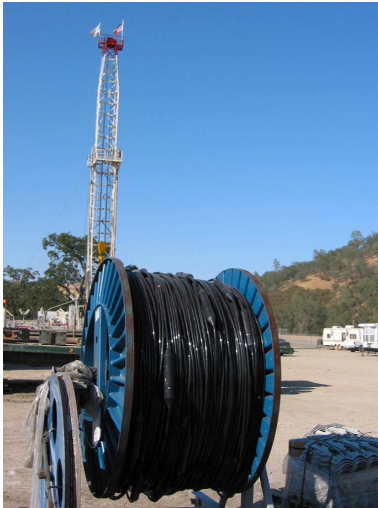
Figure 5 Downhole 240 Channel 80 Level Geophone Array
