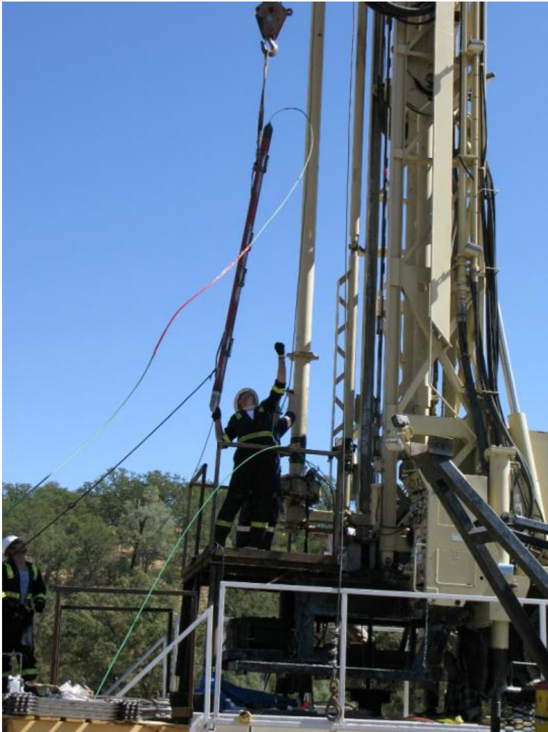
Figure 4 Installing a Pod - Control Lines are Clearly Visible
