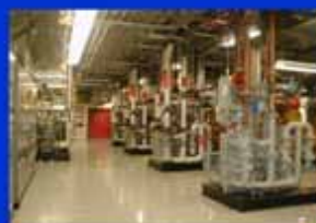
New Power Plant January 2001
