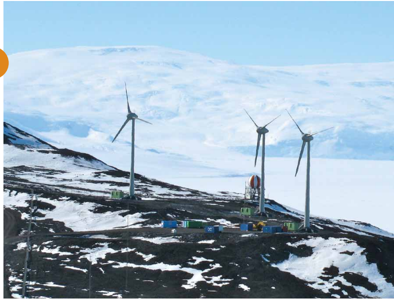
Figure 13. Wind turbines at McMurdo Station. Source: George Blaisdell.
